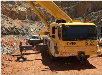
150-tonne crane to lift shaft.
