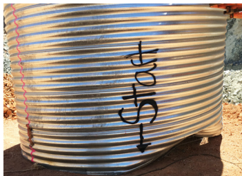
Marking doorway to match drive opening.
