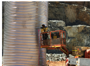
Cutting the doorway.
