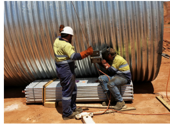
Welding lugs that would be used to suspend the first can.
