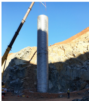
Positioning shaft over hole.
