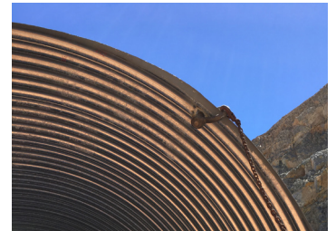
Lifting gear at top of tube.
