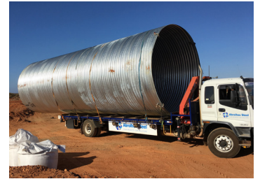
First can being taken from work zone to the pit adjacent to the raise bore.
