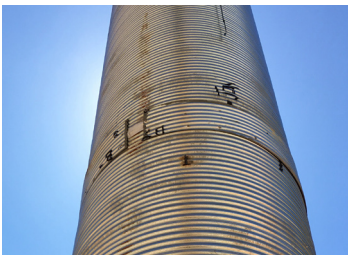
Strap joining the two tubes and ropes attached to position in drive.
