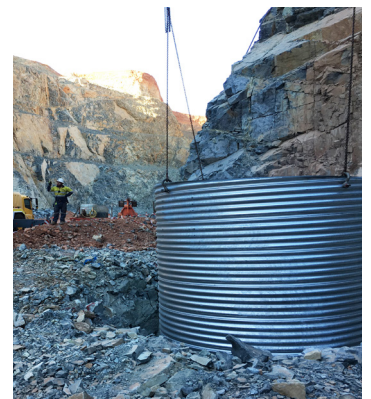
Vent shaft in final position and ready for concrete backfill.
