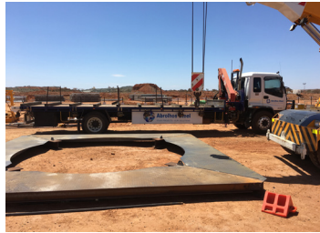
Original work platform, which was not used in construction.
