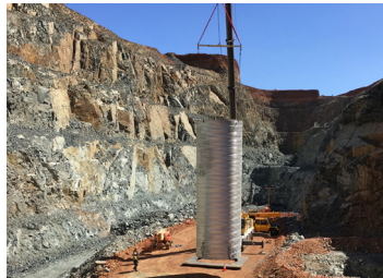
Overview in pit of work site during lift of first can.
