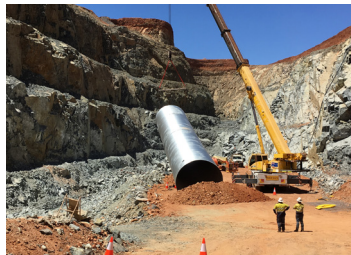
Lifting two tubes using dirt pile as a pivot.
