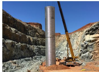
Two tubes standing together, 24m high.
