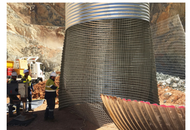
Opening cut of vent shaft.
