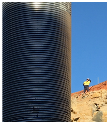
Spotter communicating with crane driver.
