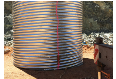
Marking opening to go into drive.
