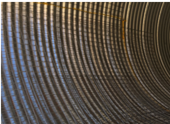
Welded mesh welded on to inside of tube.
