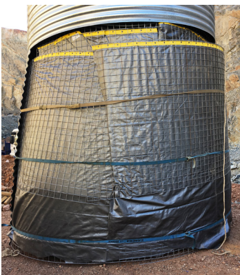
Vent bag attached to enable shotcrete at bottom of shaft.
