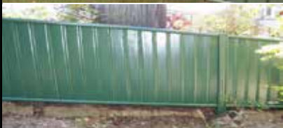
An example of a raked fence.
